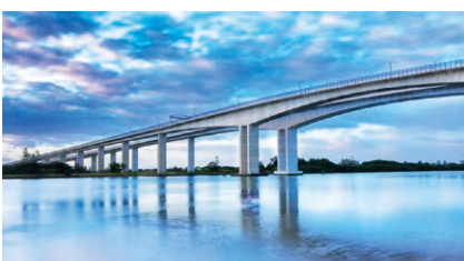
Monitor infrastructural deterioration in bridges
