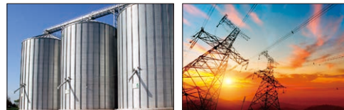
Hazardous Storage Tanks
