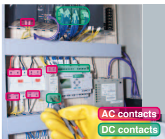
A mixture of AC and DC signals
